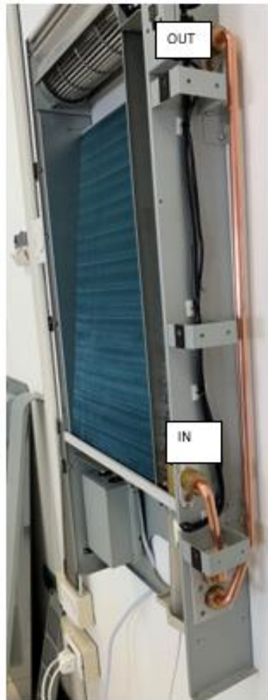
PIPE CONNECTION WITHOUT INSULATION
