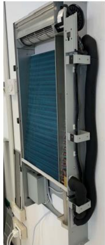
PUT INSULATION IN ALL THE EXTERNAL PIPE
