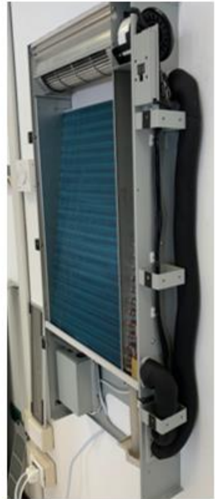
PUT INSULATION IN ALL THE EXTERNAL PIPE
